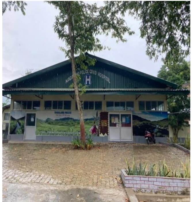
Newly constructed 70 bedded pre-fabricated COVID ward police referral hospital
